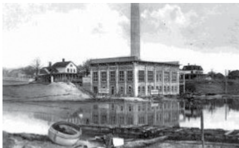
Historic Shoreline Electric Railway Powerhouse in a post card circa 1910
